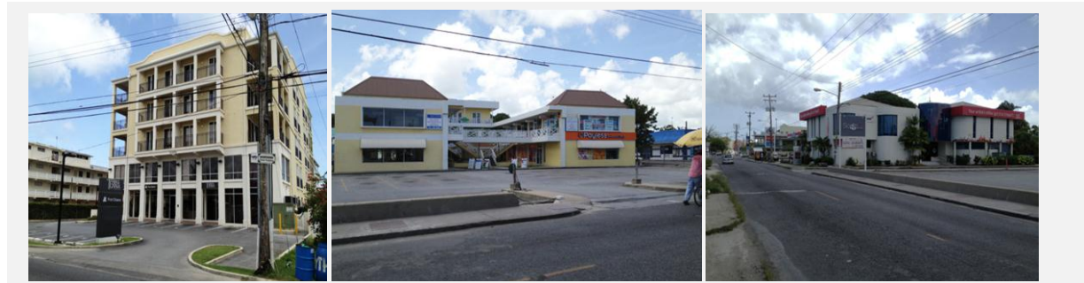
Figure 1.9. Lack of tree cover and predominance of ‘hardscape’ at various developments along the south coast’s Highway 7. The result is increased ambient temperatures and rainwater run-off, leading to a harsh, less appealing environment for patrons.
